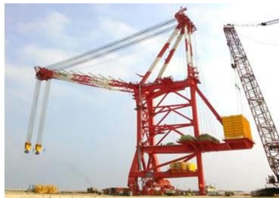
Heavy Lift Crane
